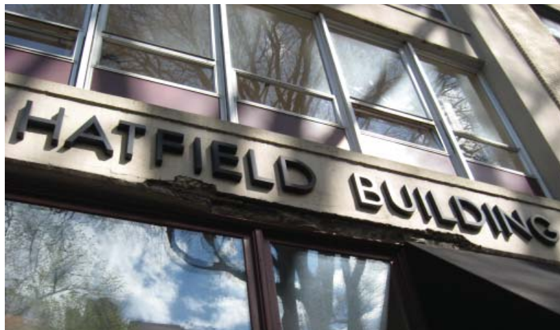
spalling concrete
